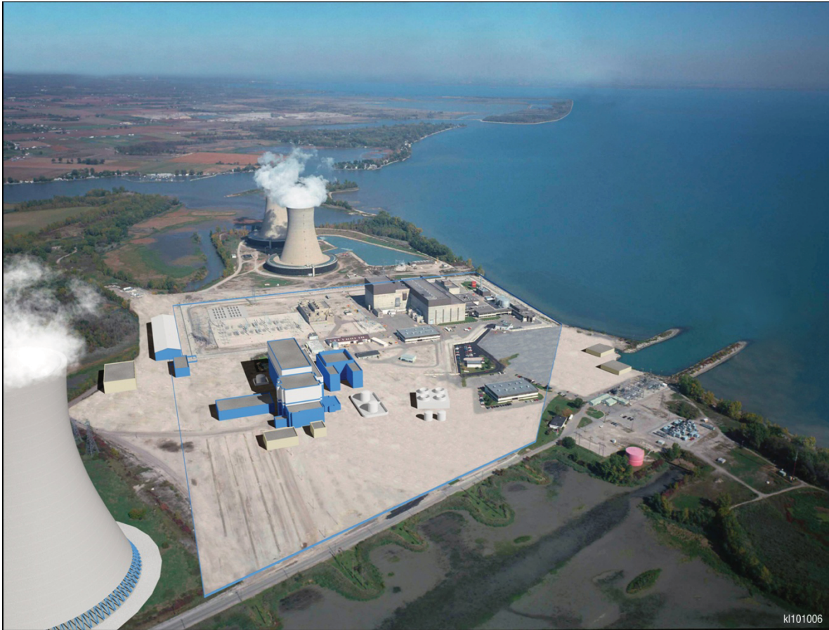
1 2 Figure 3-4. Aerial View of the Fermi Site Looking North with Proposed Fermi 3 Structures 3 Superimposed (Detroit Edison 2011b)
