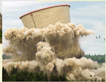
As part of the decommissioning process, the cooling tower of a nuclear power plant is imploded.
