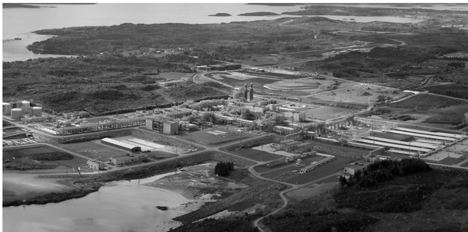
FIGURE 2 The Ormen Lange Plant on Nyhamna Island, Norway
