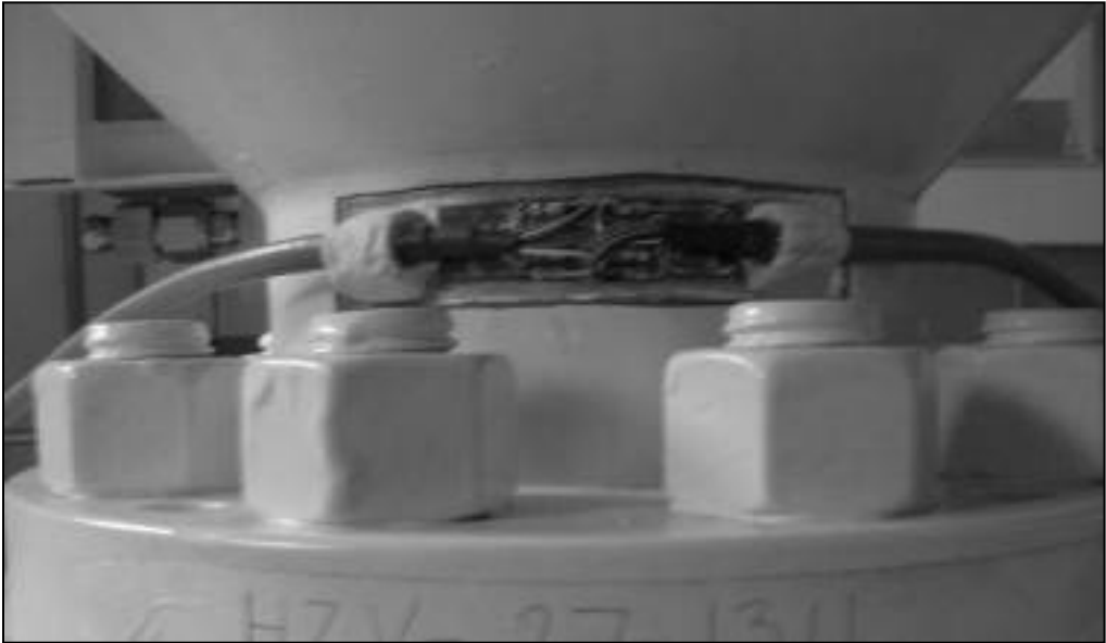
FIGURE 6 Installed Strain Gages
