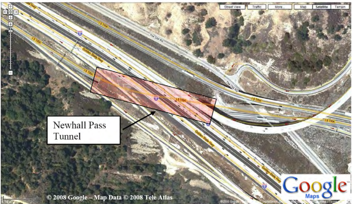
Figure 1-2. Aerial Photograph of Interstate 5 and Highway 14 Interchange. The Accident Initiated on the Exit (Southwest Side) of the Tunnel.
