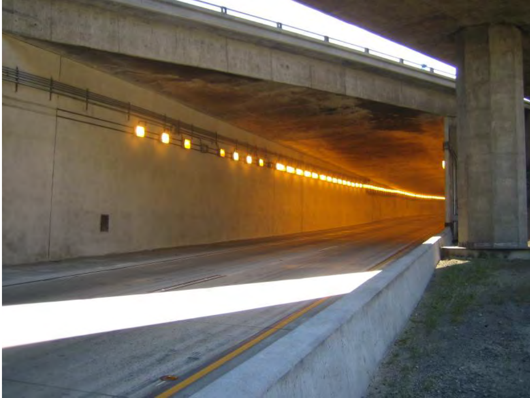
Figure 1-3. Newhall Pass Tunnel Exit After Repair
