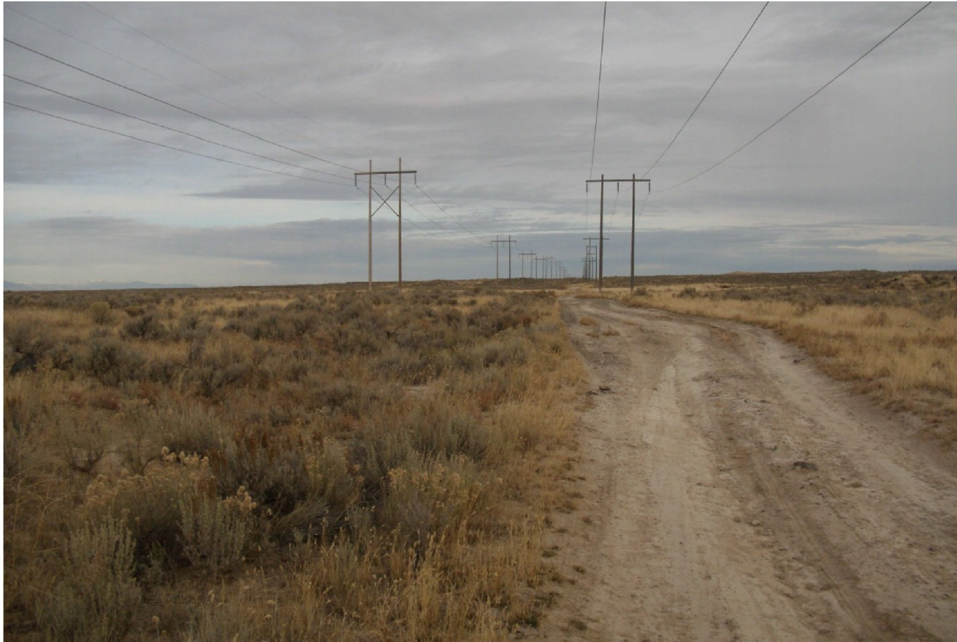
FIGURE H-5F Rev. 2 Existing Transmission Lines Along Two-Track Road on the East End of the Transmission Corridor Between the Bonneville Substation and U.S. Highway 20, Facing North EAGLE ROCK ENRICHMENT FACILITY ENVIRONMENTAL REPORT
