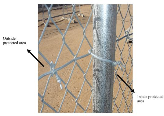
Figure 33: Example of security fence wire ties.
