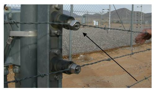
Figure 28 A tester pushes down with moderate pressure on one of the wires of a taut wire installation. Note the deflection of the switch (sensor).
