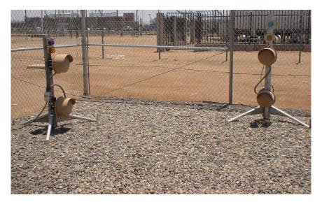
Figure 5: Example of a corner setup of microwave sensors that provides overlap to decrease the possibility of an adversary crawling beneath the beams.
