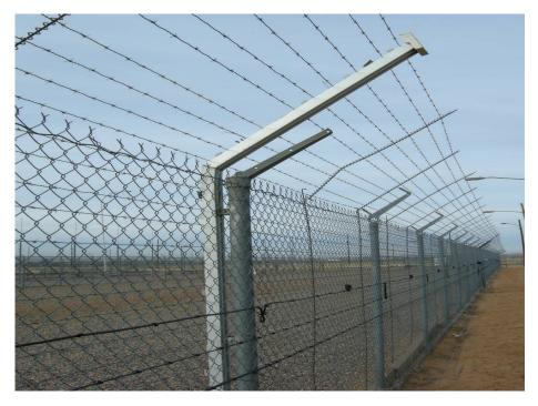
Figure 27: A taut wire sensor system installed on an existing fence. Note the application of taut wire to the outriggers in this test application.
