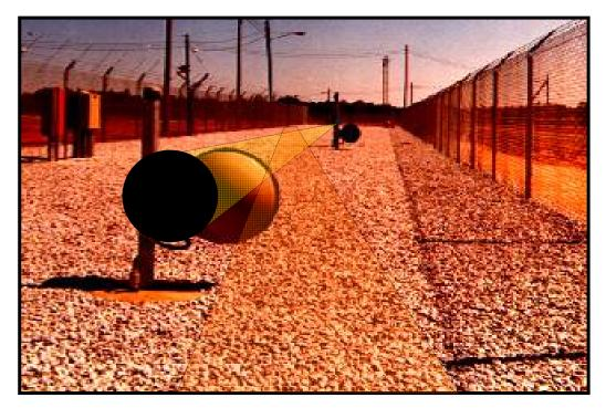
Figure 1: This photo depicts the application of microwave sensors within a perimeter intrusion detection and assessment system (PIDAS). Note that the drawn-in detection zone goes from the front microwave to another that is approximately 90+ meters (300+ feet) away. The middle microwave transmits to a unit behind the photographer. This configuration is referred to as a "basketweave" layout.
