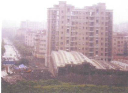
Topped Building lying flat on the ground.
