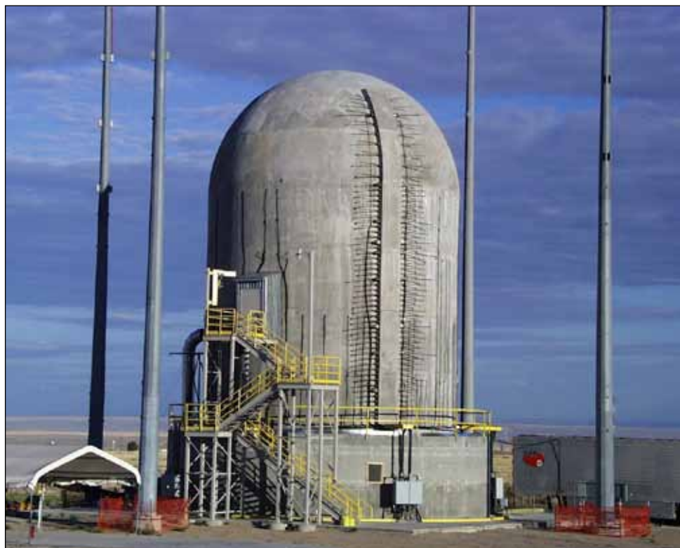
Completed prestressed concrete containment vessel 1/4-scale model at Sandia National Laboratories
