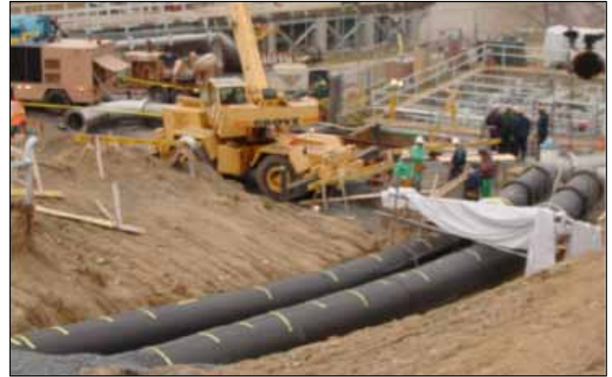
Figure 9.27 Installation of underground Class 3 safety-related HDPE piping
