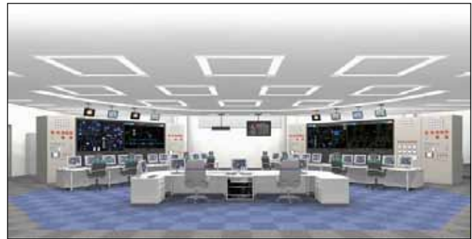
Figure 6.2 One conceptualization of an advanced control room design
