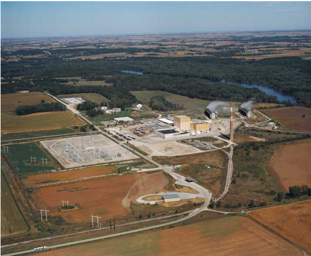
Figure 2-2. Plant Site, Switchyard, and Transmission Lines (Source: FPL-DA, 2008a)
