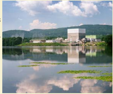
Vermont Yankee Nuclear Power Plant, located near Brattleboro, VT.
