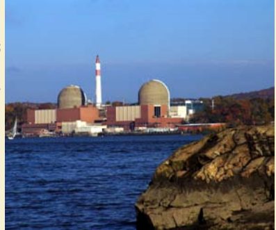
Indian Point Energy Center, located near New York City, NY.
