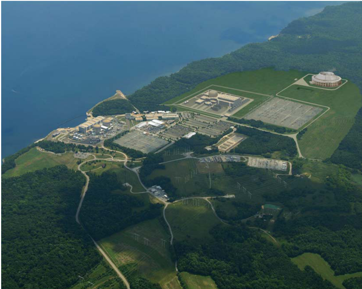
1 2 Figure 3-2. Calvert Cliffs Site with Existing Units 1 and 2 at Left and Superimposed Illustration 3 of Proposed Unit 3 at Right, Looking to the Southeast (UniStar 2009a)
