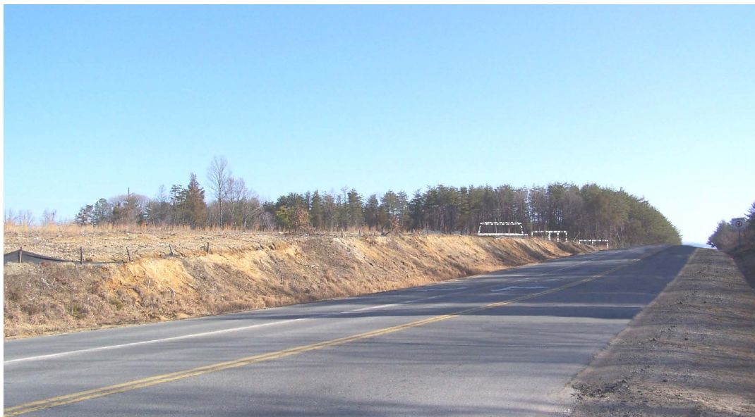
Figure 5-1. North Anna Site, Looking Northeast Along the Plant Access Road, with Outlines of Hybrid Cooling Tower (behind trees) (Source: Dominion 2009a)
