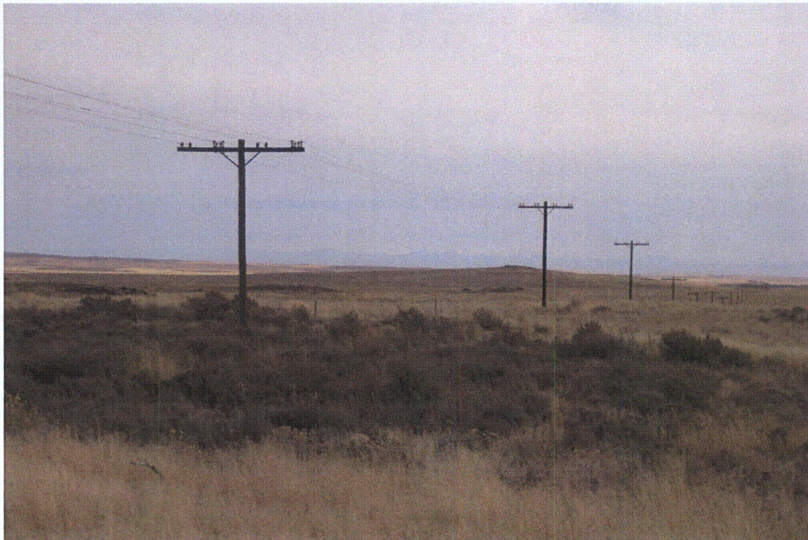
Figure H-5e. Utility lines on north side of U.S. Highway 20, facing east.
