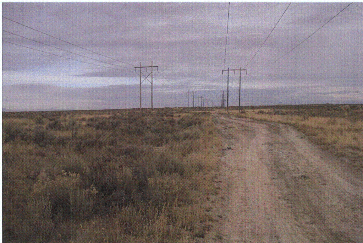
Figure H-5f Existing transmission lines along two-track road on the east end of the transmission corridor between the Bonneville Substation and U.S. Highway 20, facing north.
