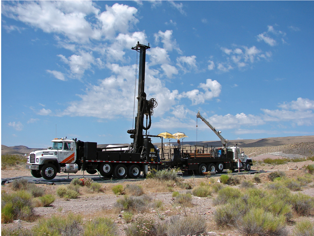
Figure 6.2-2. Typical Sonic Core Rig Operation
