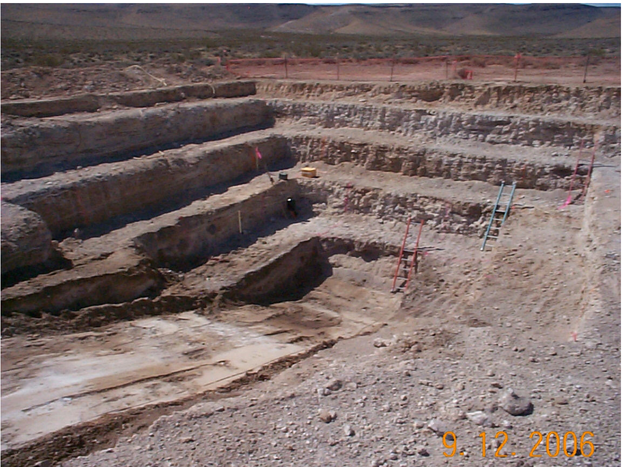
Figure 6.2-5. Test Pit #6 in the North Portal Facilities Area
