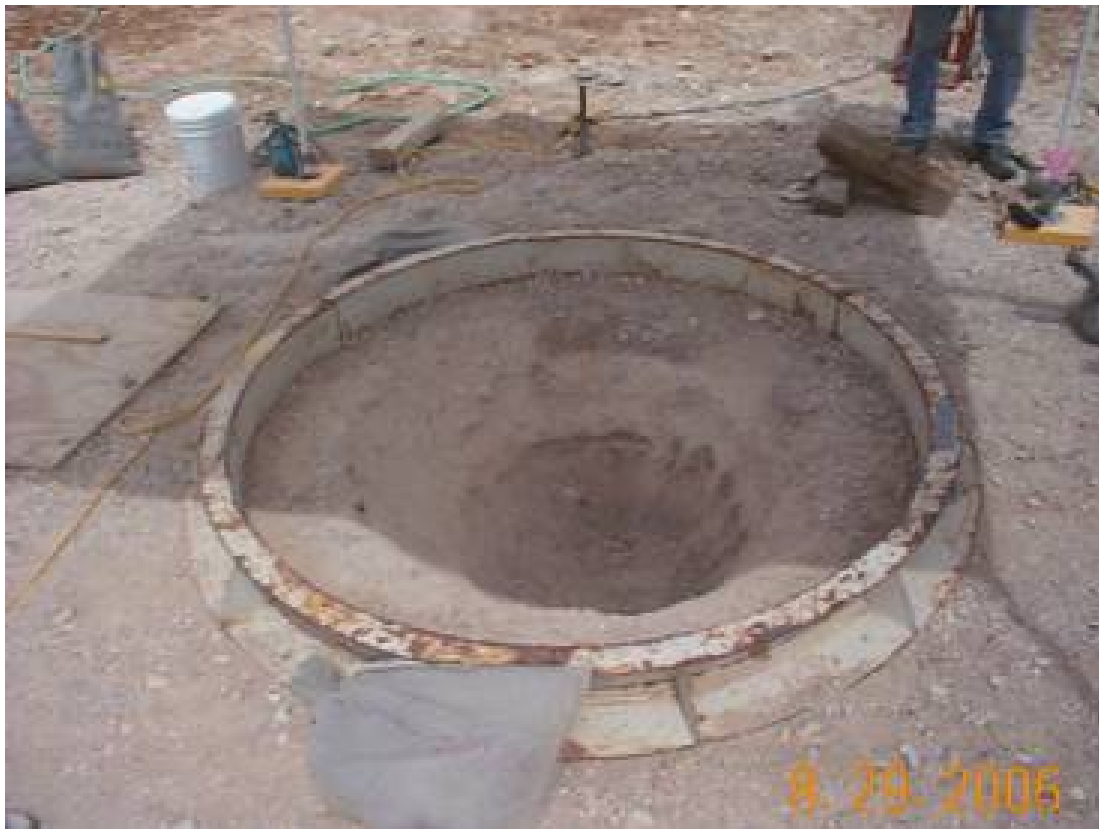
Figure 6.2-6. Ring Density Test Being Performed in a Test Pit
