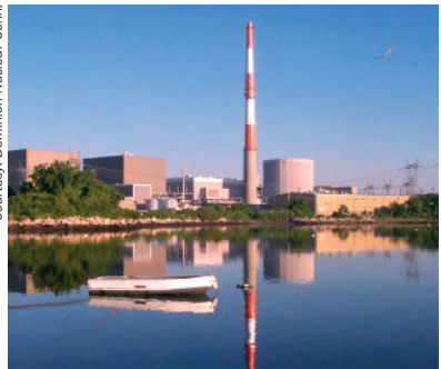
Millstone Power Station, New London, CT
