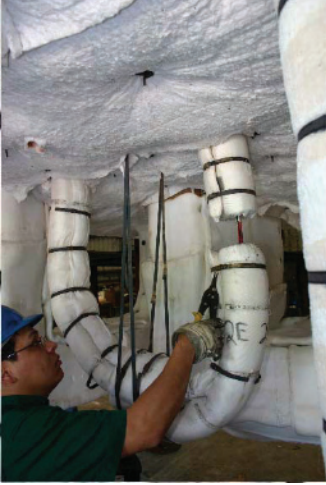
Inspection of electrical cable insulation following fire tests
