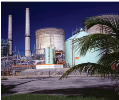
Turkey Point Nuclear Plant, Homestead, FL
