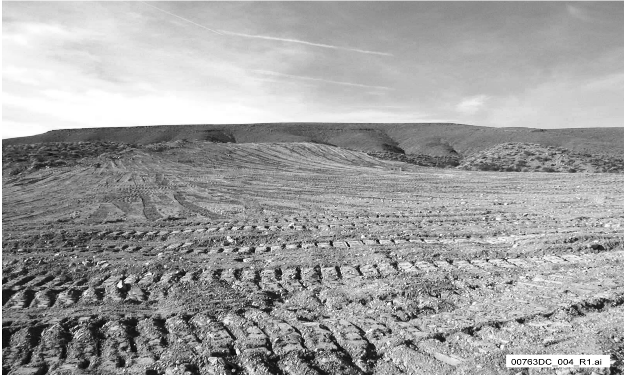
Figure 4-3. Decommissioned borrow area at Yucca Mountain that has been recontoured prior to seeding and mulching.
