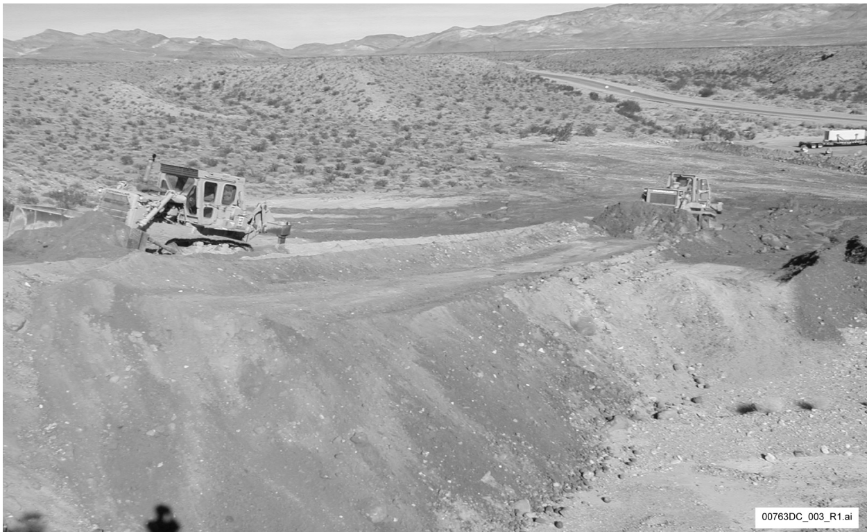
Figure 4-2. Fill material is spread and contoured on the site of a decommissioned borrow area at Yucca Mountain.
