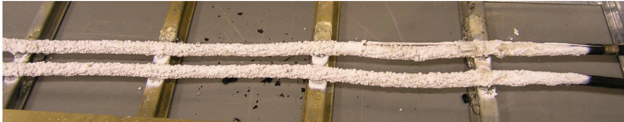
Figure 5.27: Post test photo of the SR cables following a Penlight test. Note that the cable did not fail in this test (PP-10).
