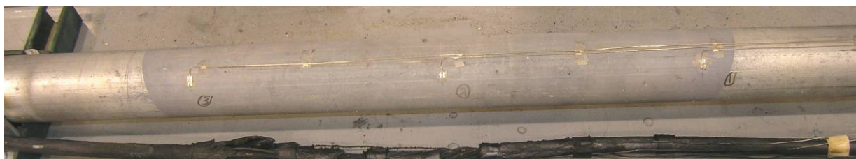
Figure 3.9: Photograph of the conduit used in Penlight showing three installed surface TCs. Note the three small bright spots along the length of the conduit with the sheathed TC leads running above each secured measurement tip and then out of the picture to the right. Each TC tip was secured to the conduit surface under a small length of stainless steel which was spot-welded to the conduit.
