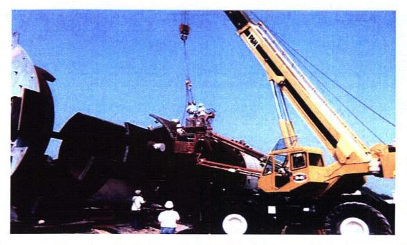
Figure 3.9 River Bend Unit 2 RPV During Disassembly
