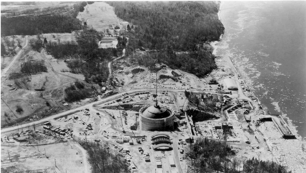
Construction of Indian Point 1
