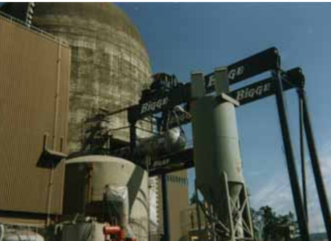
Dismantlement of a steam generator
