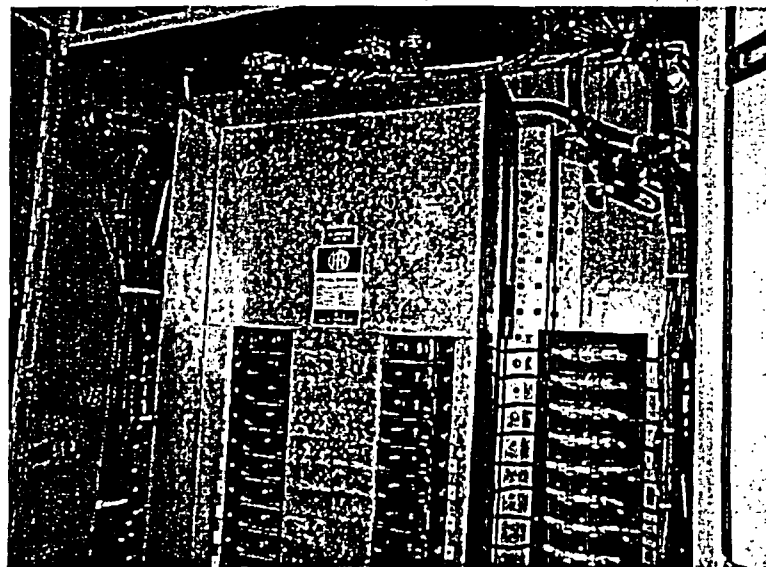
Figure G-8 Distribution Panel (Front)
