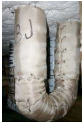
#81: 3J cable air drop complete.
