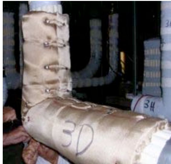
#32: Installing outer wrap on 3D LB.
