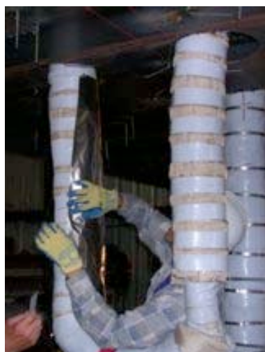
#66: Installing foil on cable air drop.
