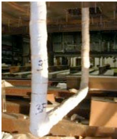
#41: Installing inner wrap on 3E.
