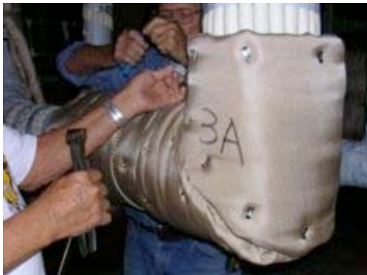
#15: Installing outer wrap on 3A.
