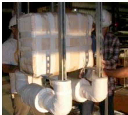
#54: 3I inner insulation.
