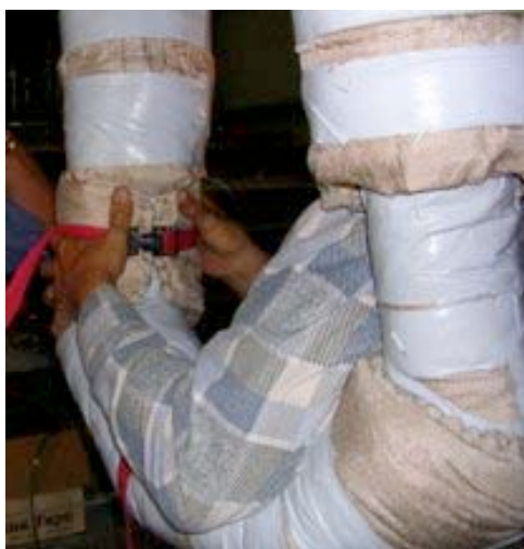
#65: 2 nd layer of insulation on air drop.
