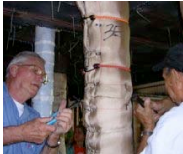
#40: Wiring outer wrap on 3E.
