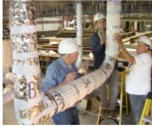
#20: Installing ATH on 3B.
