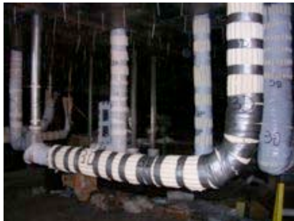
#30: ATH tubes being installed on 3D.
