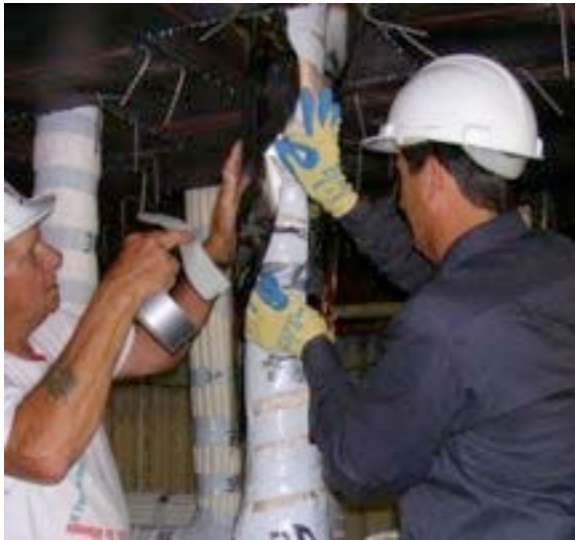
#31: Installing stainless steel foil on 3D.
