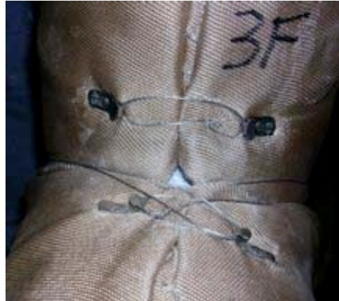
#44: Wire on inside bend of 3F LB.
