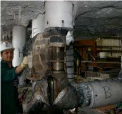
#129: 3B opened to expose LB and conduit.
