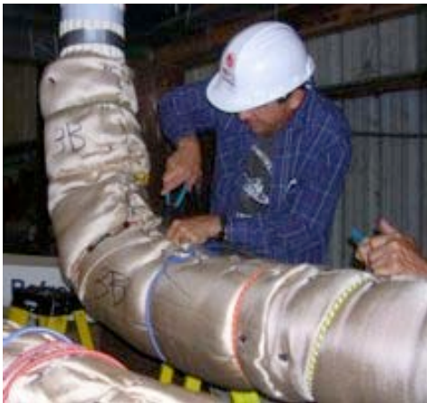
#23: Wrapping elbow on 3B.
