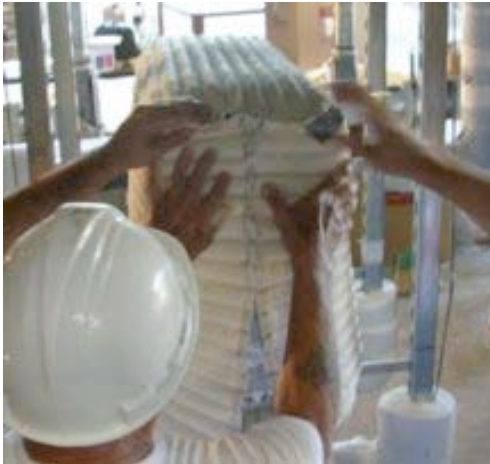
#57: Installing ATH on junction box.
