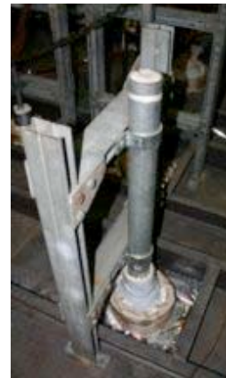
#88: Conduit seal on cold side.
