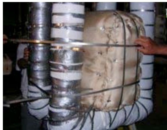
#60: Installing support bands on JB.
