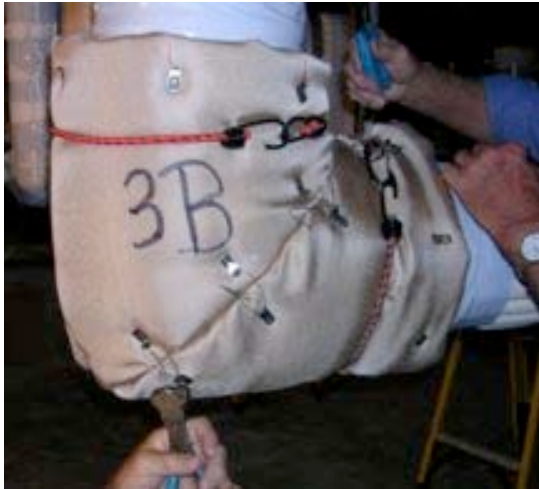
#21: Installing outer wrap on 3B LB.
