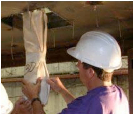
#29: Installing inner insulation on 3D.
