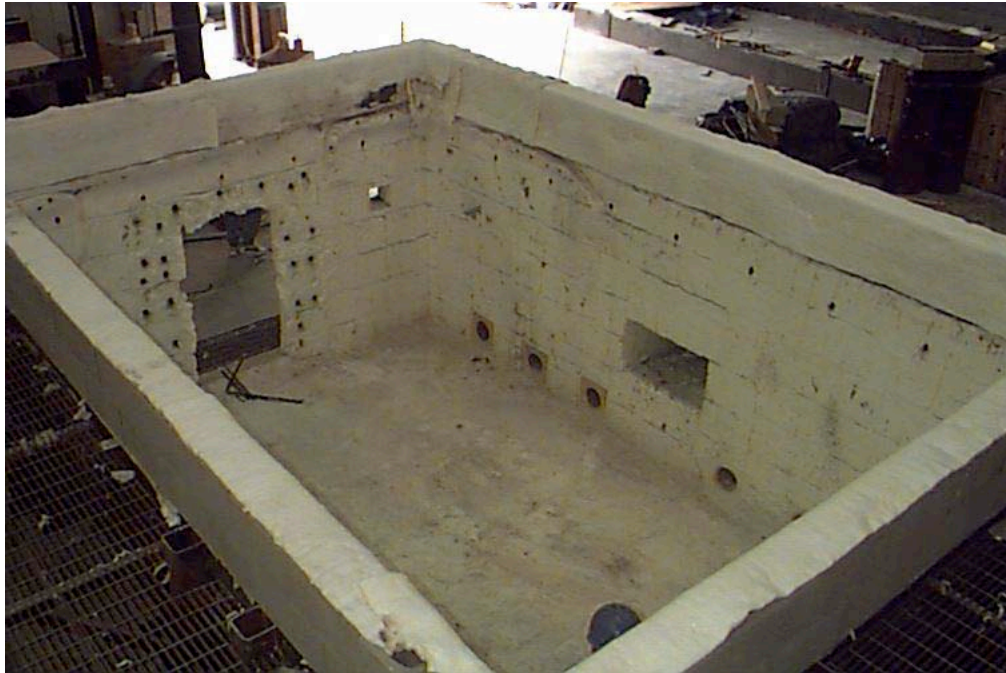
12' x 18' Horizontal Furnace (Overhead View)
