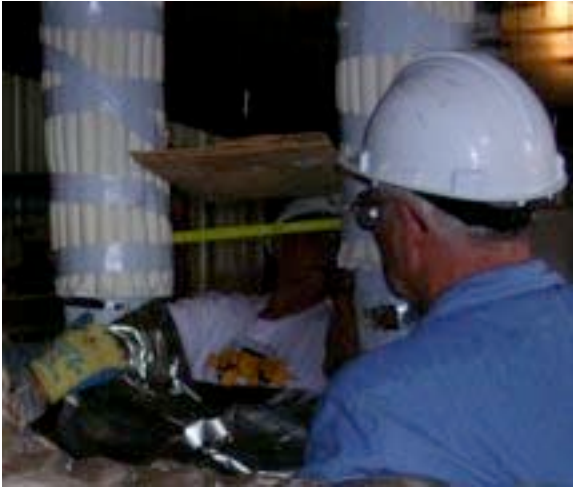
#67: Installing ATH tubes on air drop.
