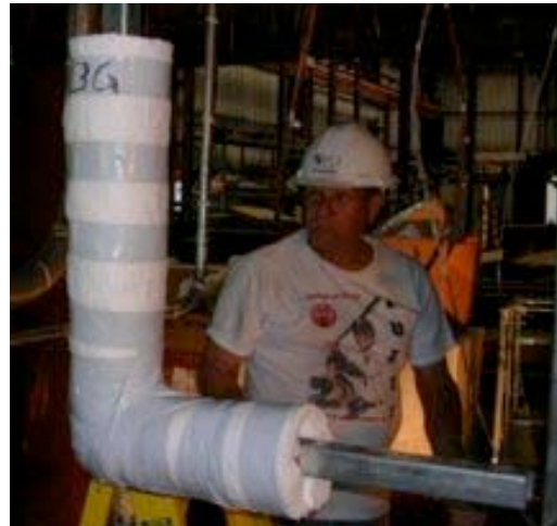
#46: Installing inner wrap on 3G.
