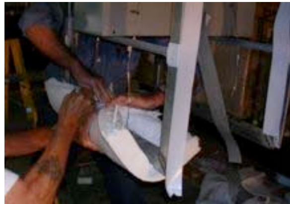
#52: Wrapping supports on 3I junction box.
