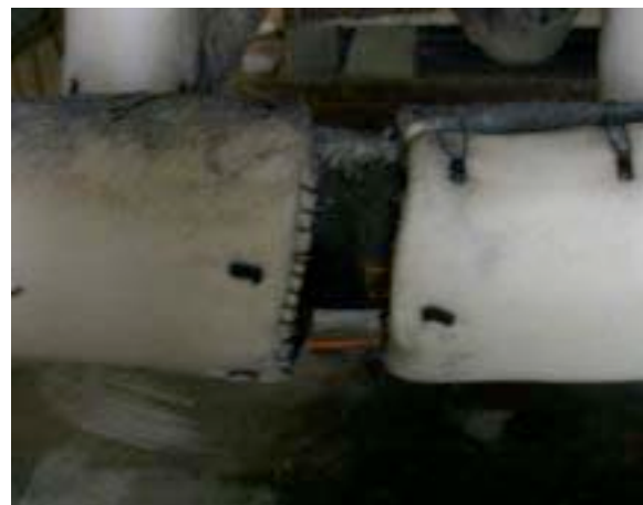
#126: Gap in 3C to foil (typical).
