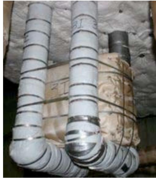
#80: 3I (junction box) complete.
