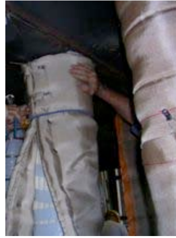
#68: Installing outer insulation on air drop.
