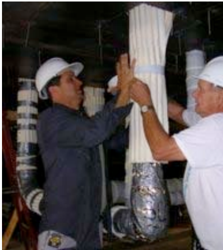
#27: Applying ATH tubes to 3C.
