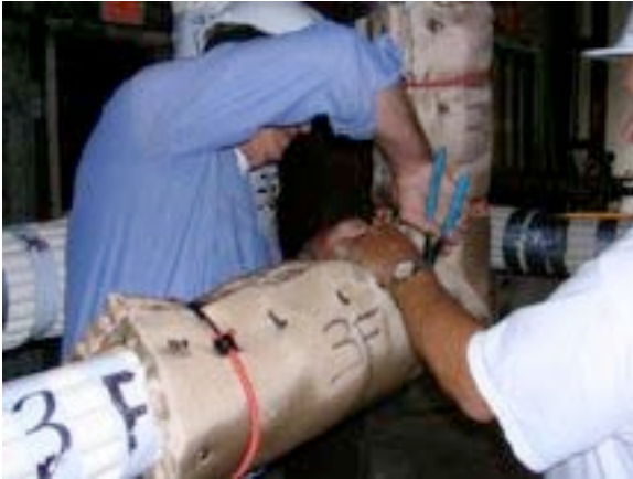
#43: Installing outer wrap on 3F LB.
