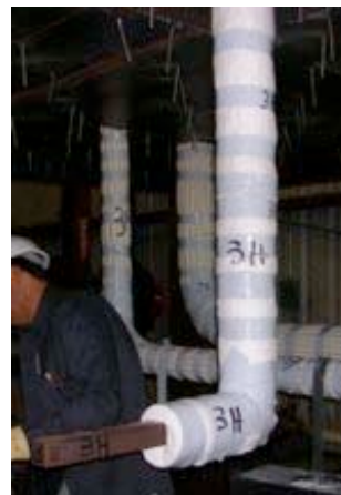
#48: Inner insulation on 3H.
