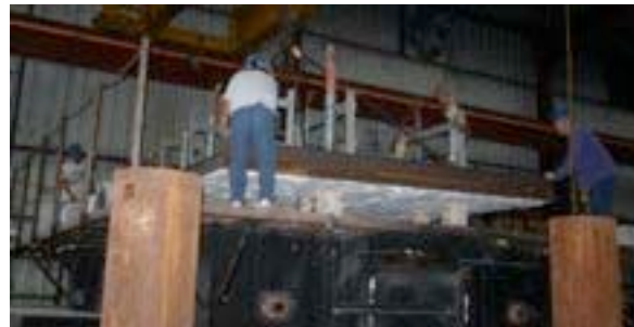
#84: Lowering assembly onto furnace.
