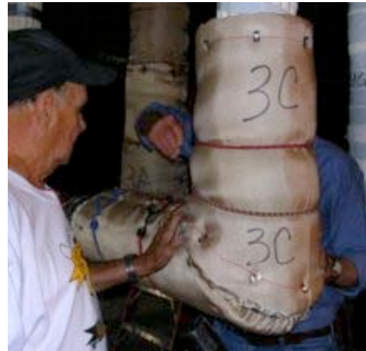
#28: Installing outer wrap on 3C.
