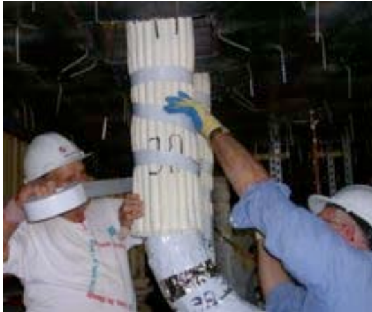
#13: Installing ATH on 3A.
