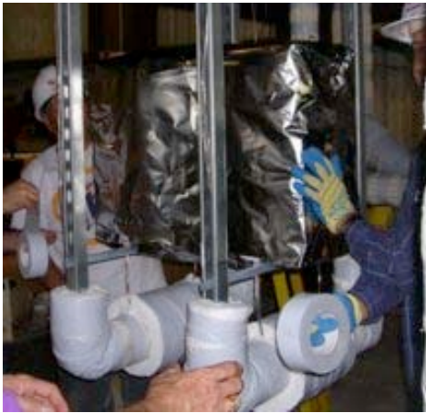
#55: Installing stainless steel foil on junction box.
