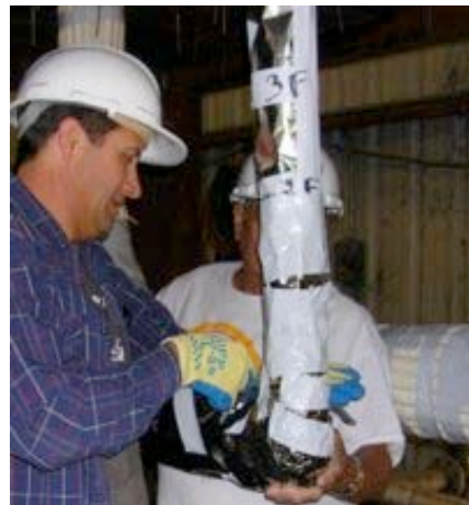
#42: Installing foil on 3E.
