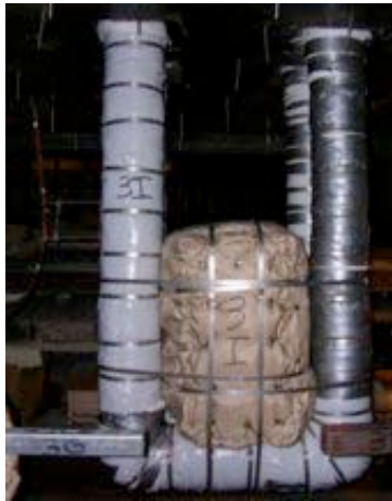
#61: Junction box installed.
