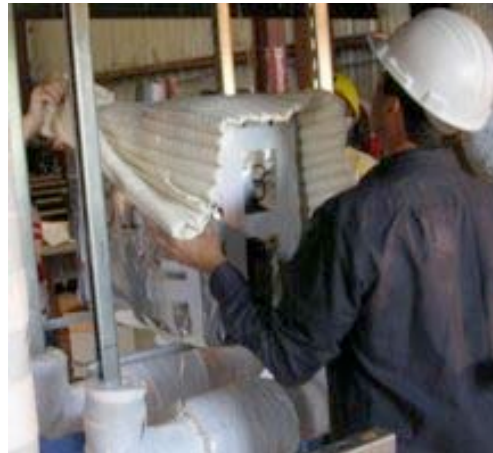
#56: Installing ATH on junction box.
