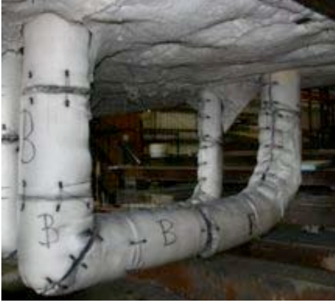
#115: Item 3B after hose stream test.
