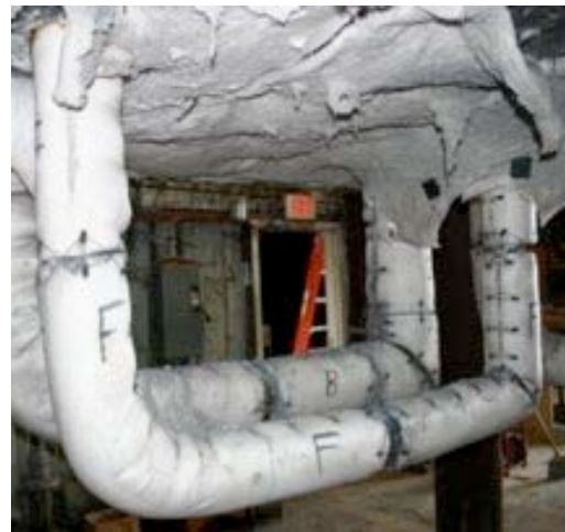
#120: Item F after hose stream test.
