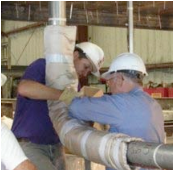
#11: Installing wrap on 3A elbow.
