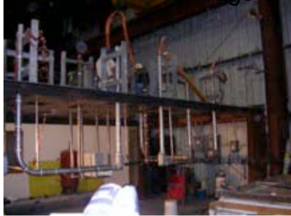
#2: Test items installed in deck.
