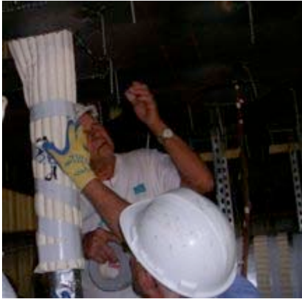
#37: Installing ATH on 3E.
