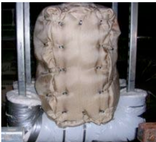
#59: Installing outer wrap on JB.
