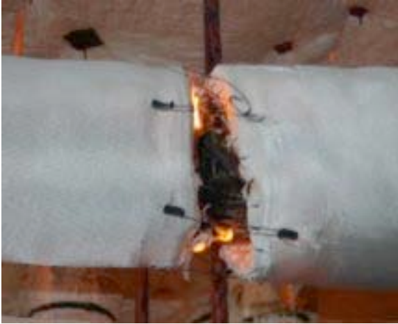
#97: Typical gap between outer layer blankets.
