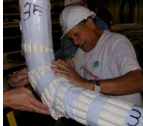
#38: Installing ATH on 3E.
