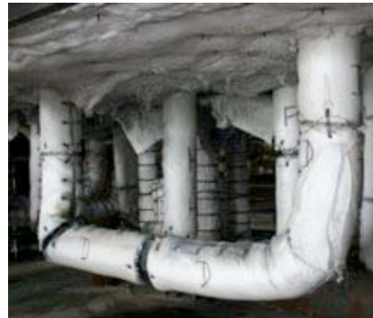
#118: Item 3D after hose stream test.
