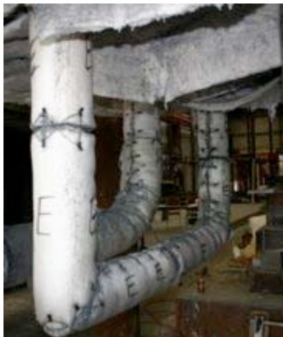
#119: Item 3E after hose stream test.
