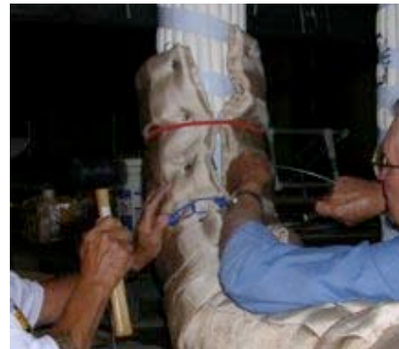
#16: Wiring outer wrap on 3A.
