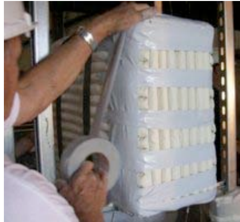
#58: Taping ATH tubes on junction box.
