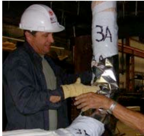
#12: Installing foil on 3A elbow.
