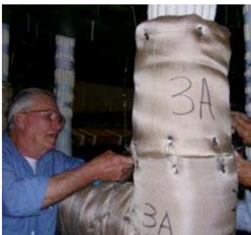
#17: Completing wrap on 3A.
