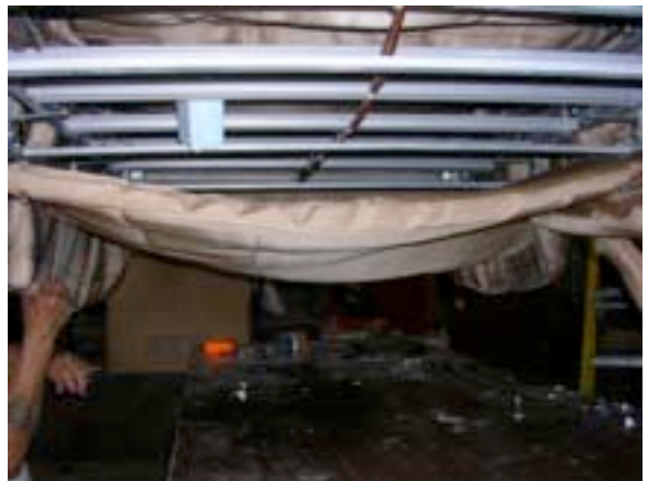
#40: 2D bottom pad installation.
