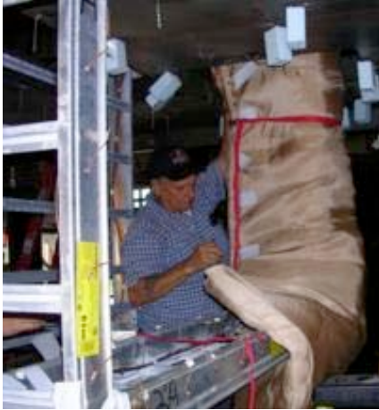
#13: Installing wrap on 2A.
