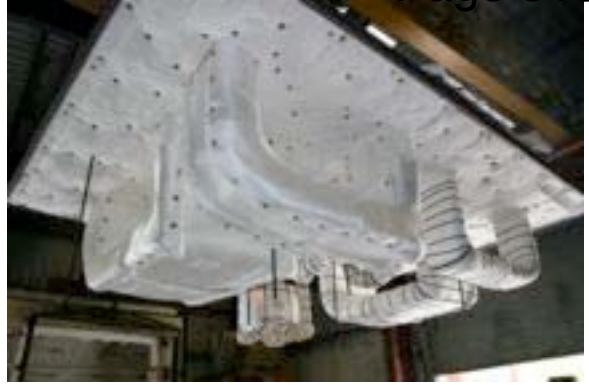
#98: Specimen after fire exposure.
