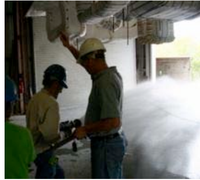
#106: Adjusting nozzle for hose stream test.
