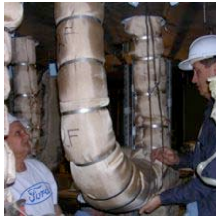
#54: Installing center support bands on 2F.
