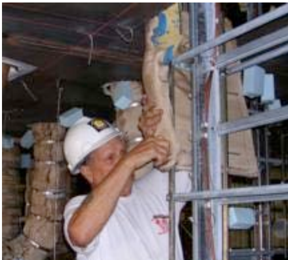
#35: Installing side pad on 2D.
