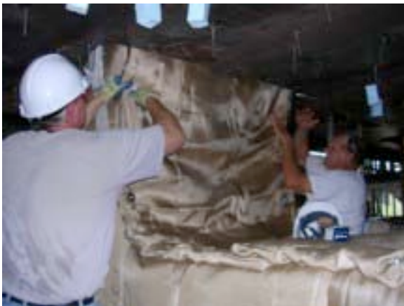
#39: Installing to pad on 2D.
