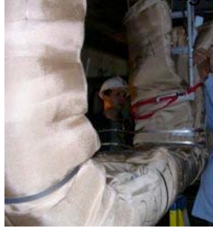
#14: Completing 2A wrap.
