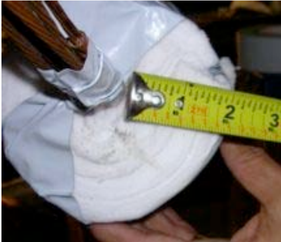
#49: Verification of 2" thickness.
