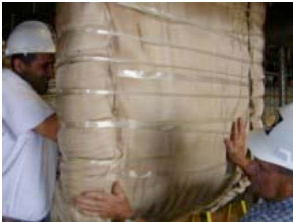
#29: Cladding 2C elbow back.
