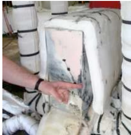
#136: showing wrinkled steel.
