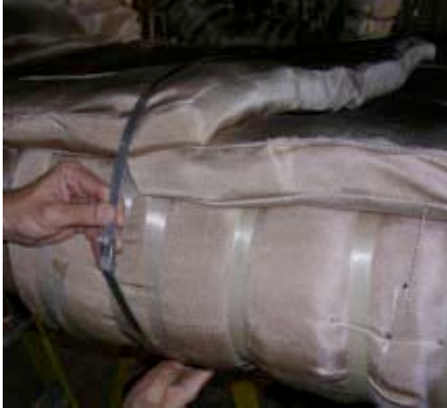
#31: Banding pads at overlap (2C).
