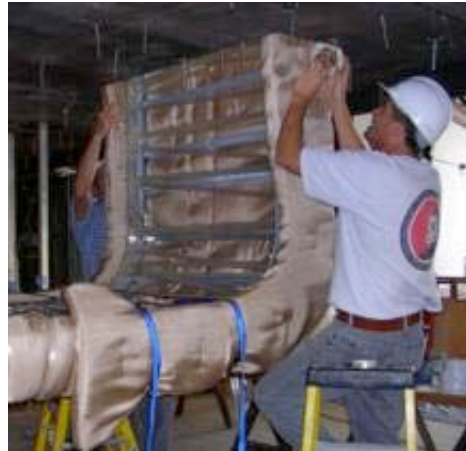
#28: Cladding 2C elbow sides.
