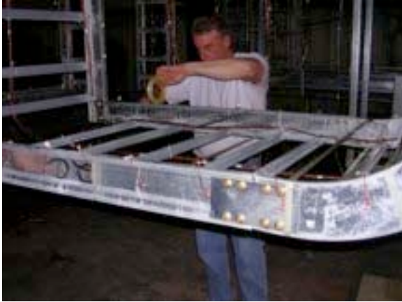
#7: Item 2C installing support tape.
