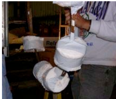
#48: Installing 2" stand-offs on item 2F.
