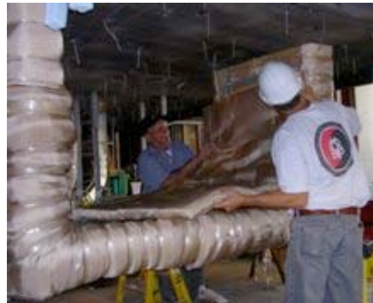
#30: Installing 2C top pad.
