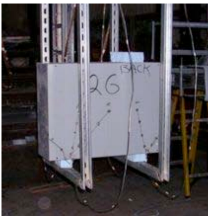
#11: Junction box ready for cladding.
