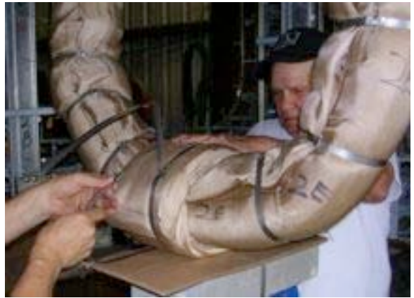
#46: Banding 2E center joint cover.
