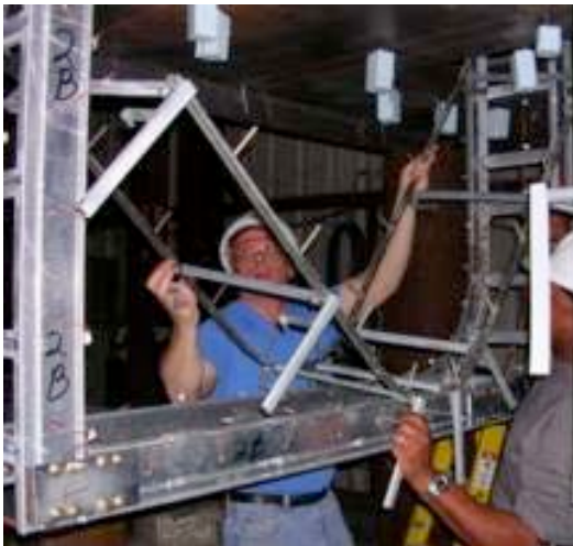
#5: Item 2B installing 2" air gap.
