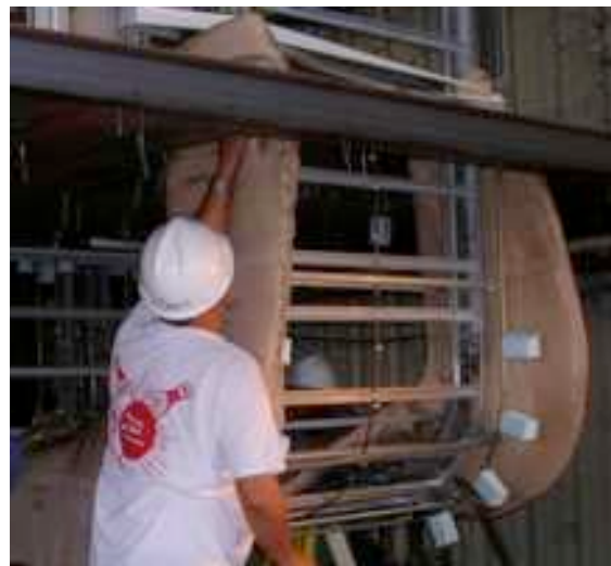
#36: Installing side pads on 2D.
