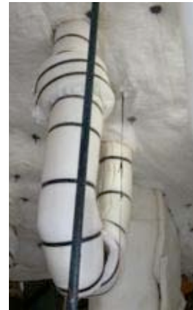
#120: Item 2F after hose stream test.
