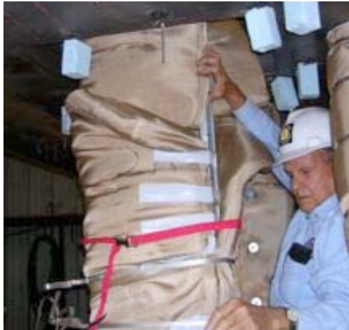
#15: 2A wrap extending through deck.
