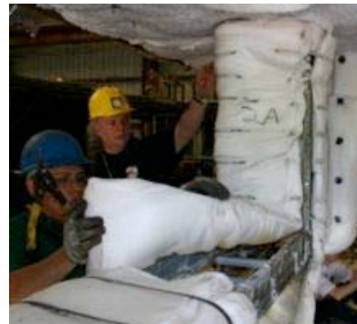
#126: Item 2A being disassembled.
