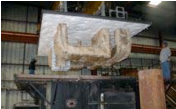
#83: Placing assembly on furnace.
