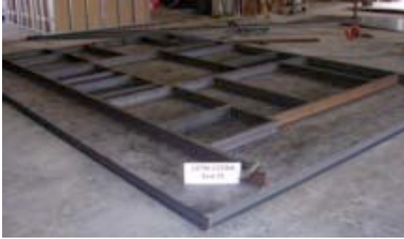
#1: Test deck under construction.
