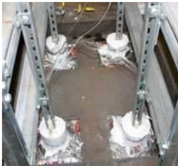
#87: Top side of Junction Box supports.
