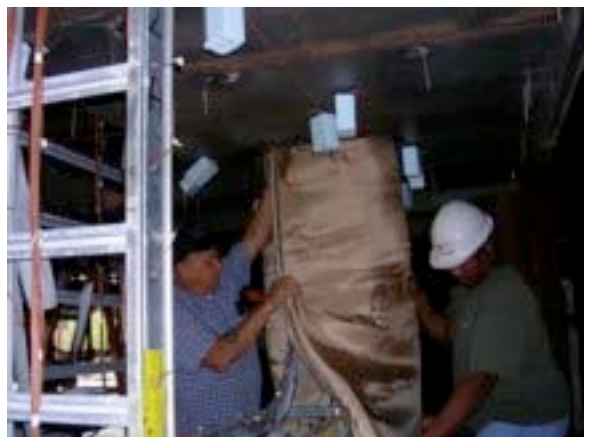
#12: Item 2A direct wrap installation.
