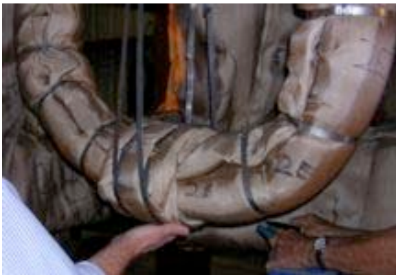
#47: Installing 2E center support bands.
