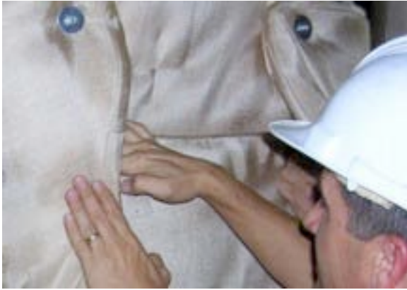
#19: Item 2B bolt connections.
