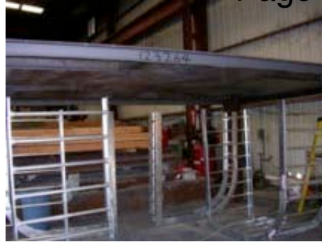
#2: Trays ready to install in deck.
