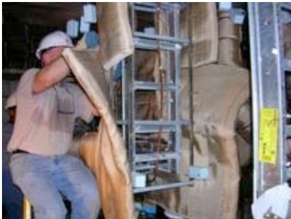
#17: Wrapping of 2B started.
