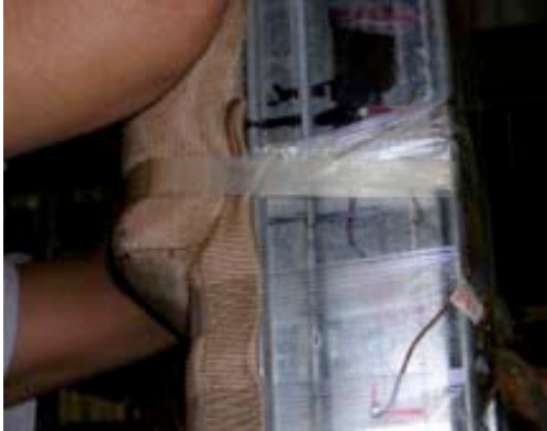
#25: 3" overlap on joints (Item 2C).
