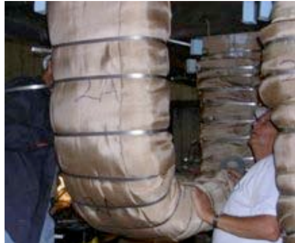
#16: 2A banding completed.
