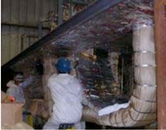
#67: Insulating the steel deck.
