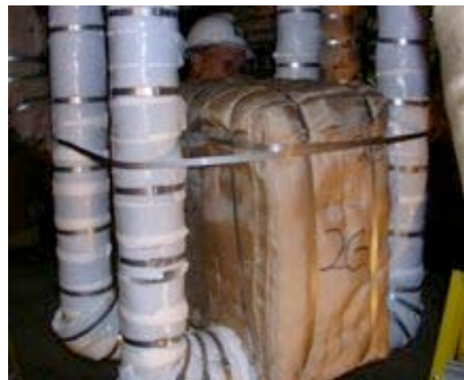
#66: Applying final bands on JB.
