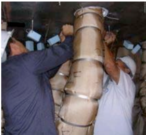
#53: Installing bands on 2F.
