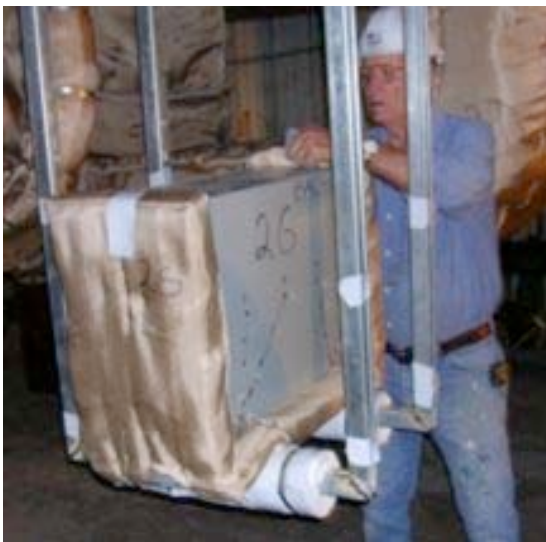
#59: Wrapping junction box.
