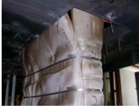
#32: Wrapping through deck penetration.
