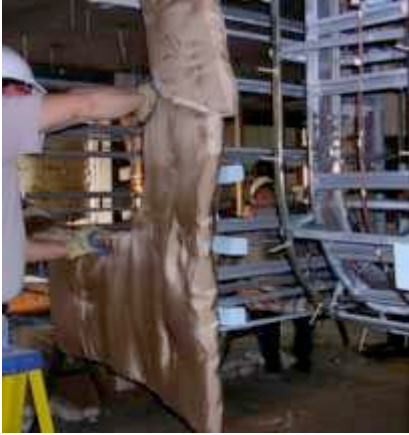
#37: Installing side pad on corner.
