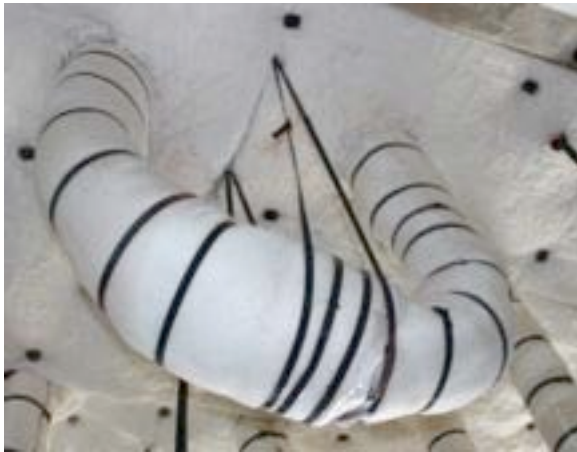
#119: Item 2E after hose stream test.
