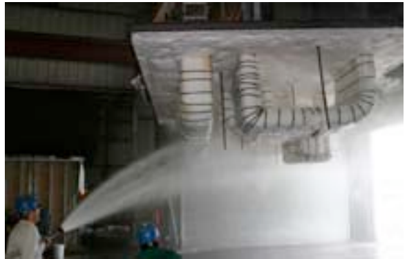
#108: Hose stream test.
