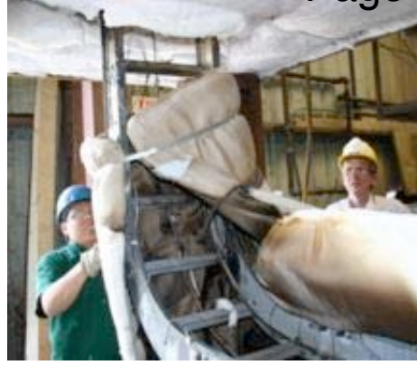
#128: Item 2A elbow end being unwrapped.
