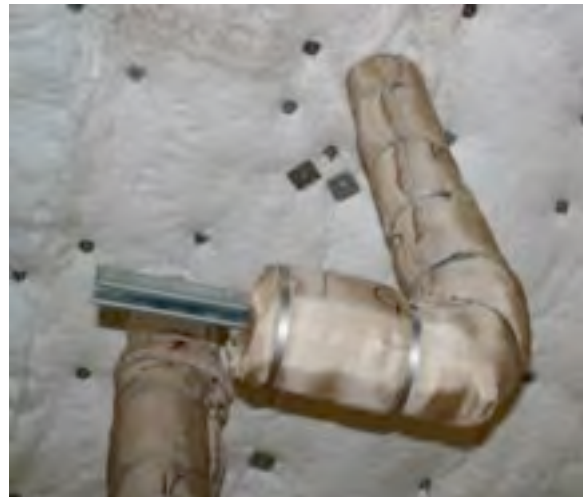
#66: Support 1G completed.
