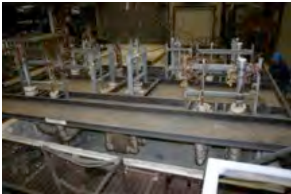
#75: Lowering onto furnace.
