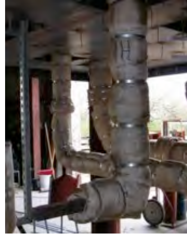
#50: Support 1H completed.
