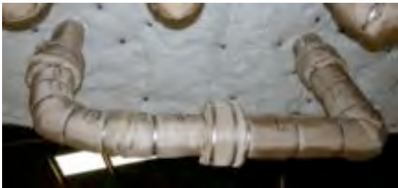
#65: Bottom view of conduit 1D.
