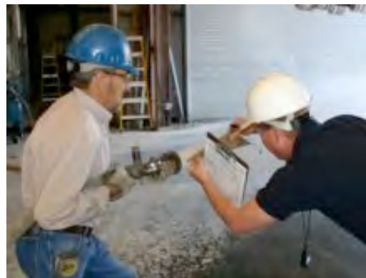
#114: Adjusting nozzle flow.
