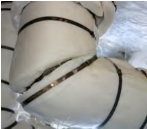
#141: Conduit 1B joint at LB.
