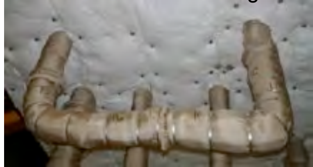
#62: Conduit 1C completed.
