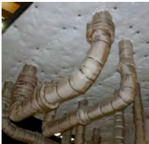
#59: Conduits 1B & 1F completed.
