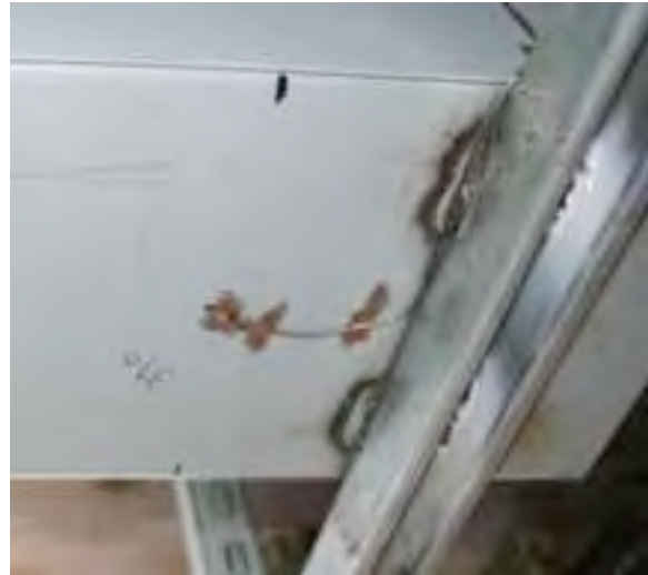
#22: JB attachment welds.
