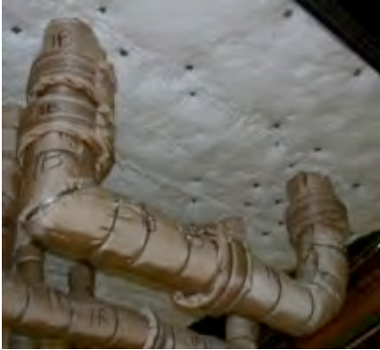
#61: Conduit 1B completed.
