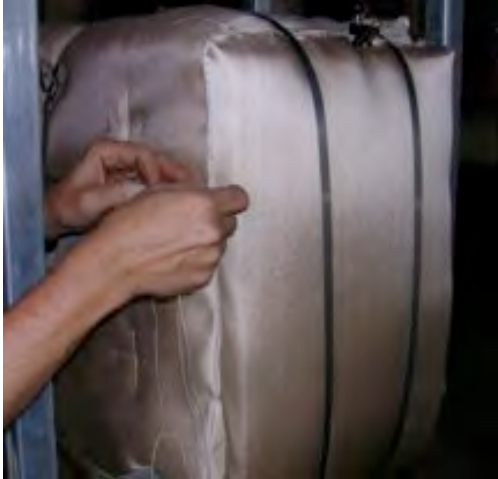
#55: Stitching seams on JB insulation.
