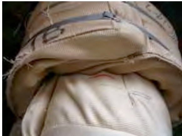
#34: Conduit 1B joint cover.
