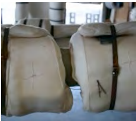
#137: Gap on 1A with collar removed.
