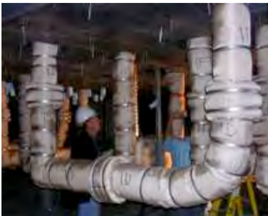
#41: Conduit 1D completed.
