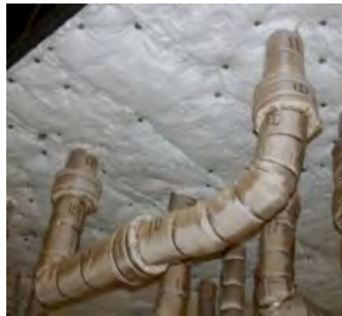
#64: Conduit 1D completed.
