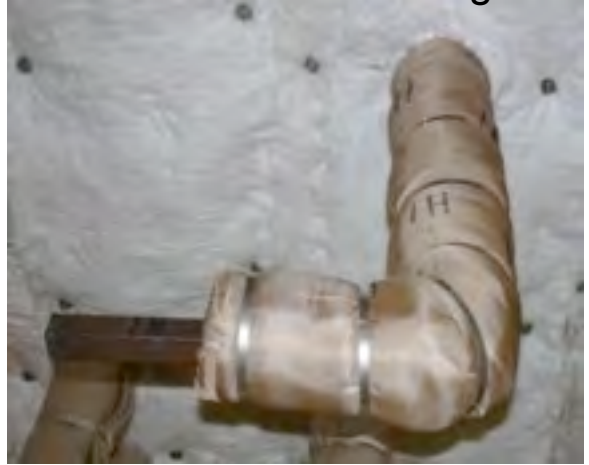
#68: Support 1H completed.
