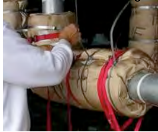
#32: Cladding the LB on conduit 1B.
