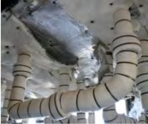
#133: Conduit 1D after hose stream.
