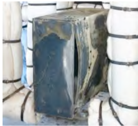
#132: JB with insulation removed.
