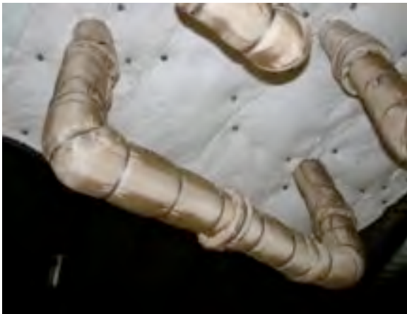
#63: Conduit 1C completed.
