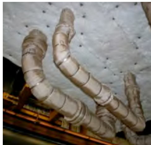
#60: Conduits 1B & 1F completed.
