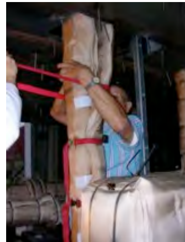
#54: Cladding JB supports.
