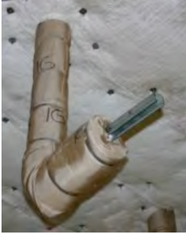
#67: Support 1G completed.
