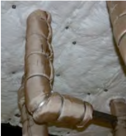
#69: Support 1H completed.
