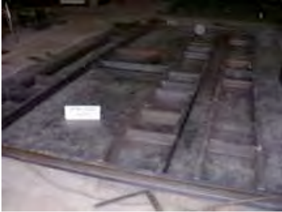
#1: Deck under construction.
