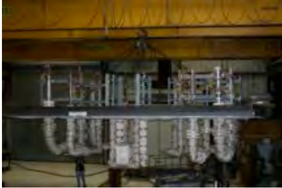
#73: Lowering onto furnace.
