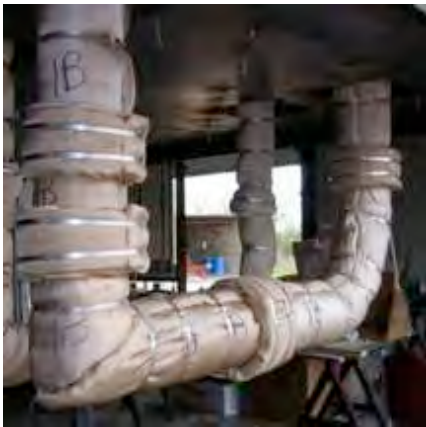
#33: Conduit 1B completed.
