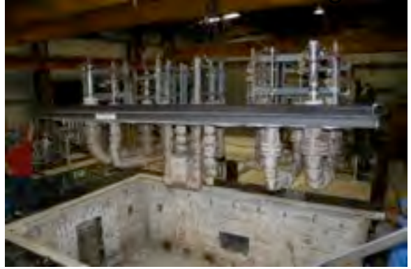
#74: Lowering onto furnace.
