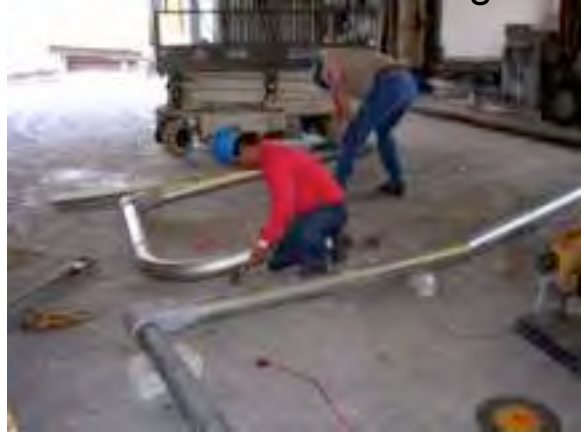
#2: Assembling conduits.
