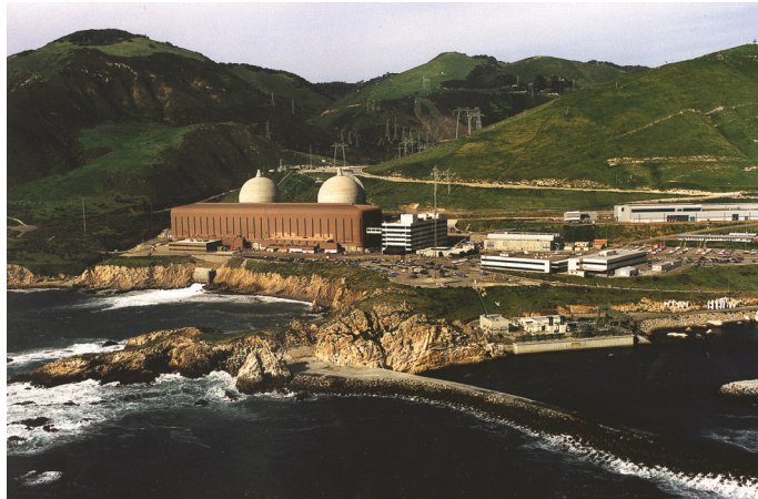
Diablo Canyon, Nuclear Power Plant
