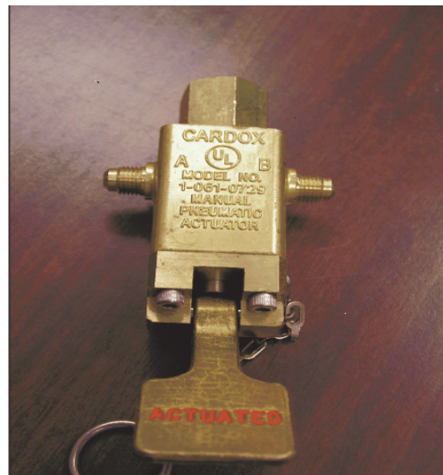
Figure 1 - Manual-Pneumatic Actuator
