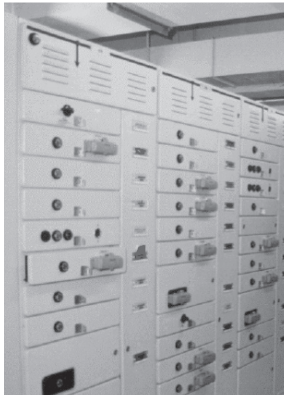
Figure 4: Switchgear equipped current transformers inside the plug-in unit and with diagnosis sockets for adaptation of the external SIPLUG®
