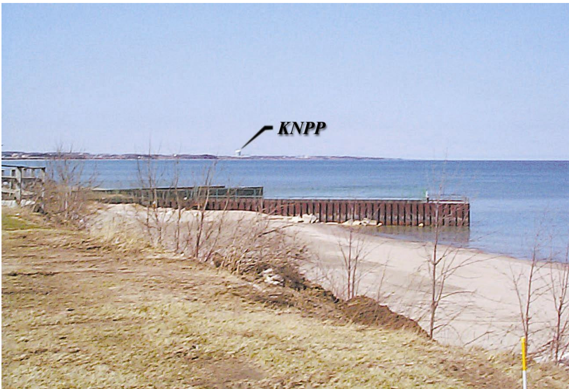
View of Kewaunee Nuclear Power Plant from PBNP
