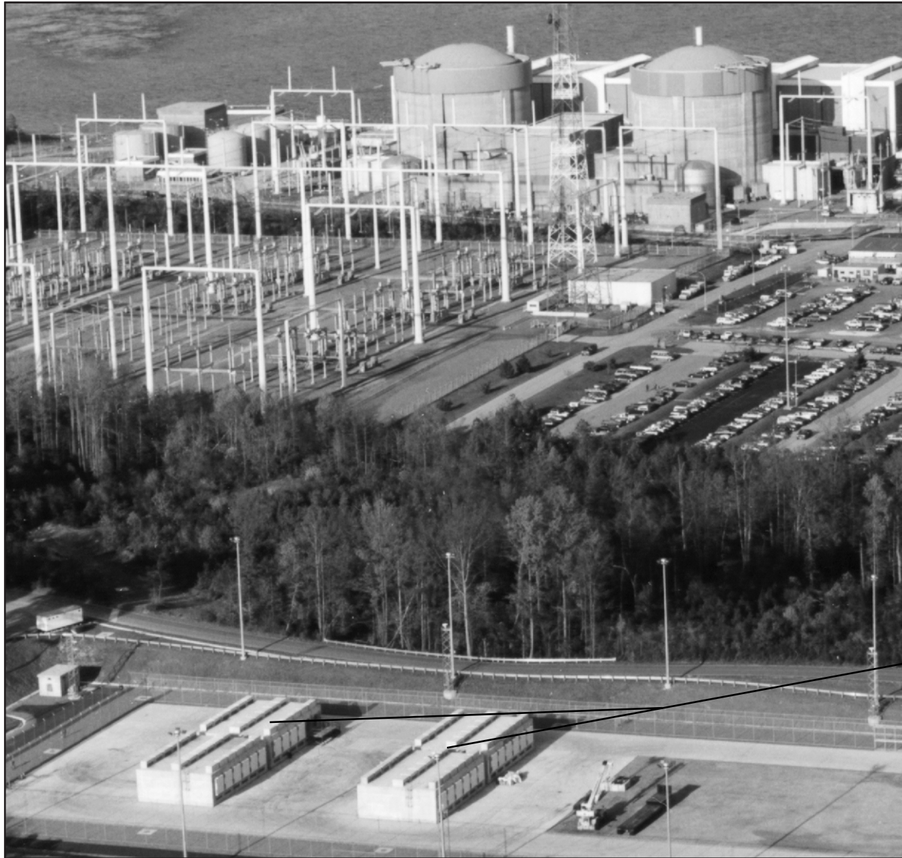
Figure 7-2. Typical independent spent fuel storage installation.
