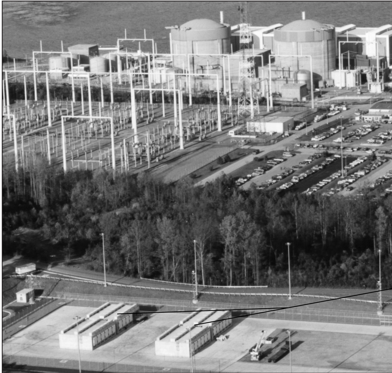
Figure 2-32. Typical independent spent fuel storage installation.
