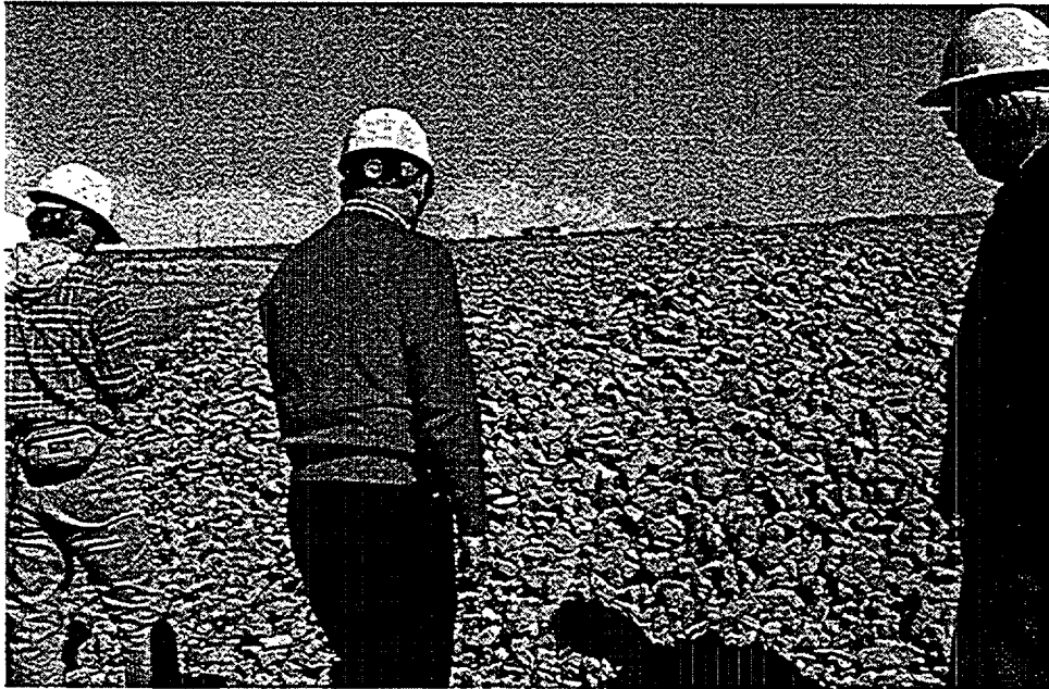
Figure F-3. Marginally-placed riprap.
