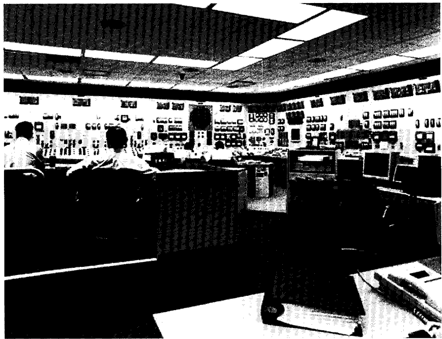
Control Room at a Nuclear Power Plant
