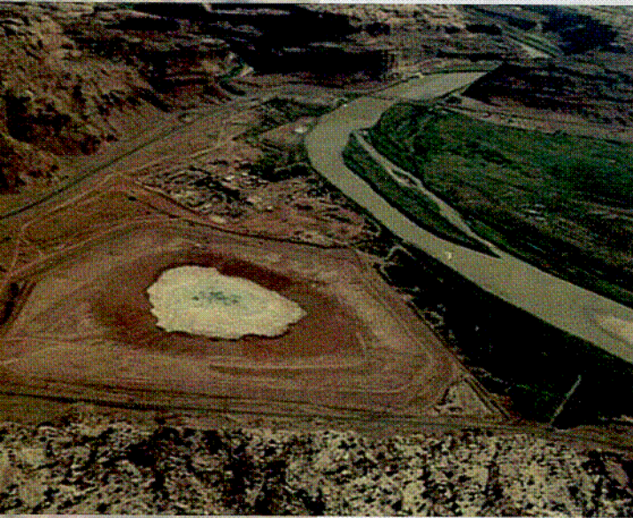
Aerial view of Atlas mill tailings site near Moab, Utah, with Colorado River in background
