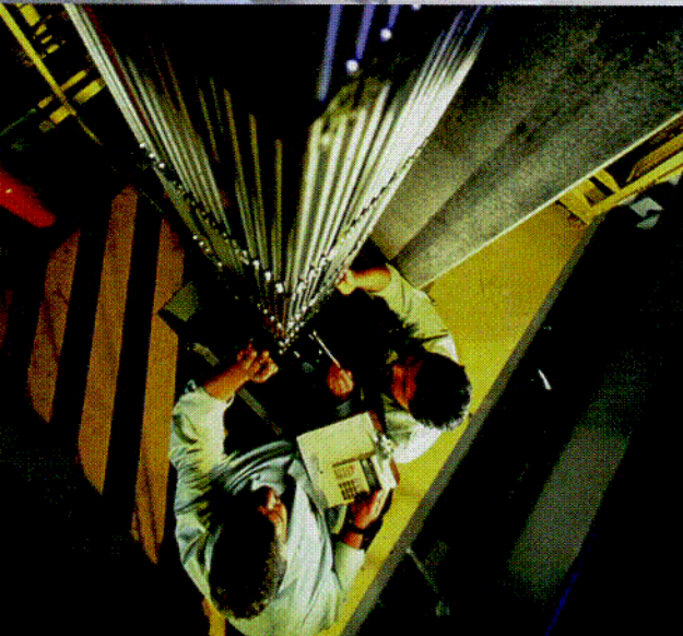
Photo courtesy of Siemens Power Corporation.
