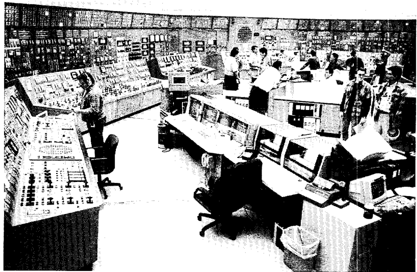
Control Room at a Nuclear Reactor
