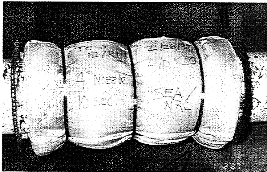
Figure 3-13. Target blanket installation.
