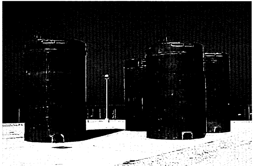
Independent Spent Fuel Storage Casks
